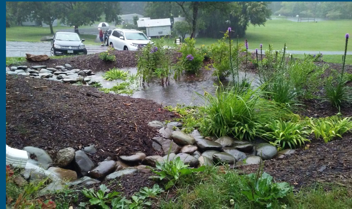
Fully installed rain garden in use, demonstrates ponding of water.
