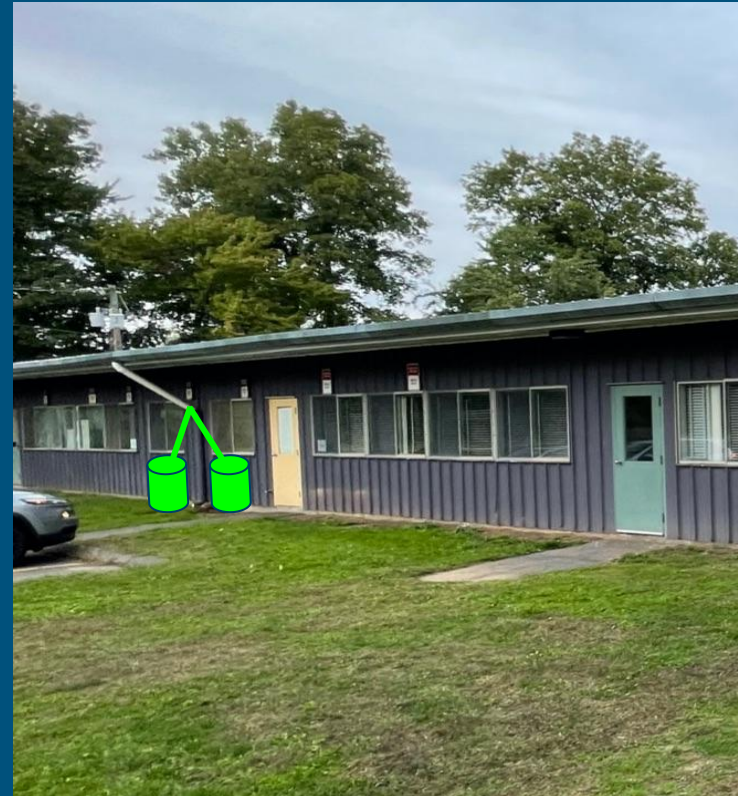
Conard High School Ground Image - Reach Program Building Side View
