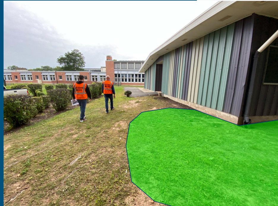
Conard High School Ground Image, Reach Program Building - rain garden number one
