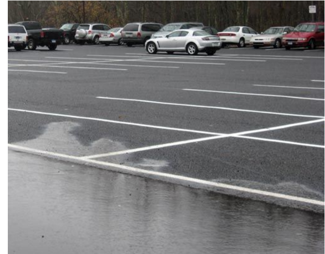
Water flowing off of impervious asphalt into pervious asphalt
