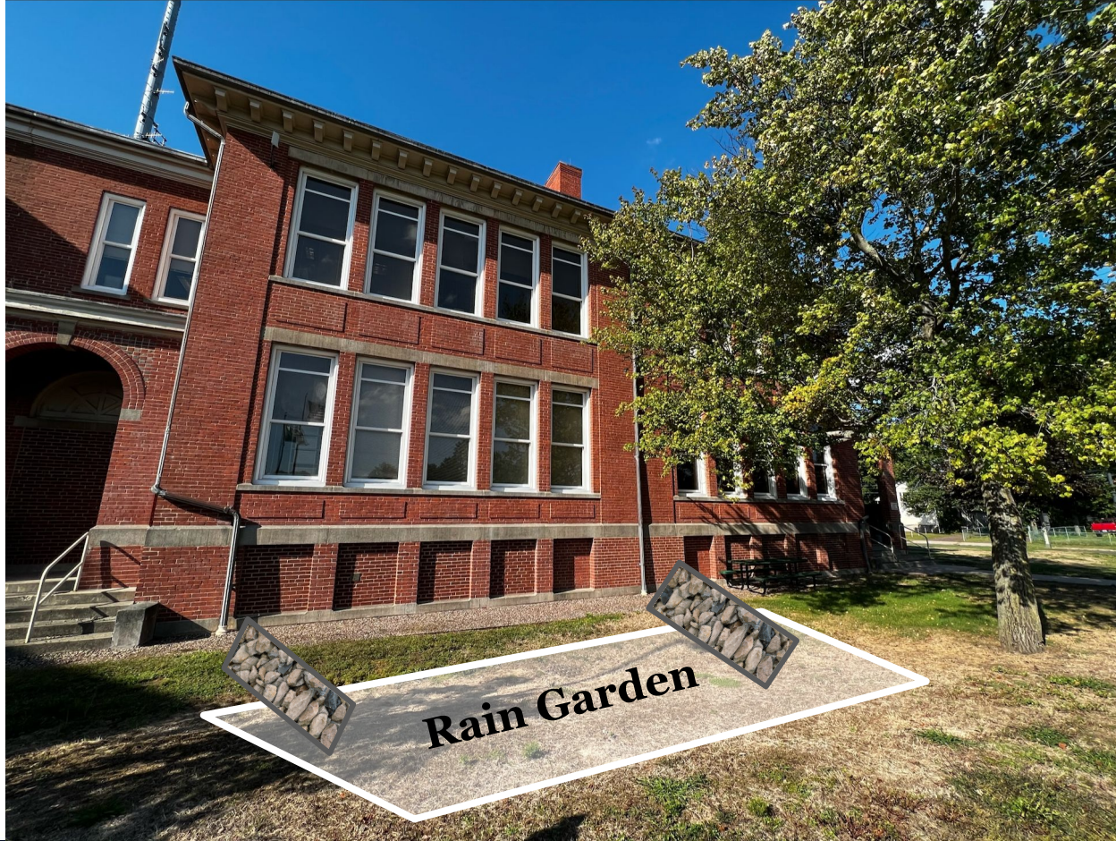
Project #6: Rain Garden at the Public Safety Complex
