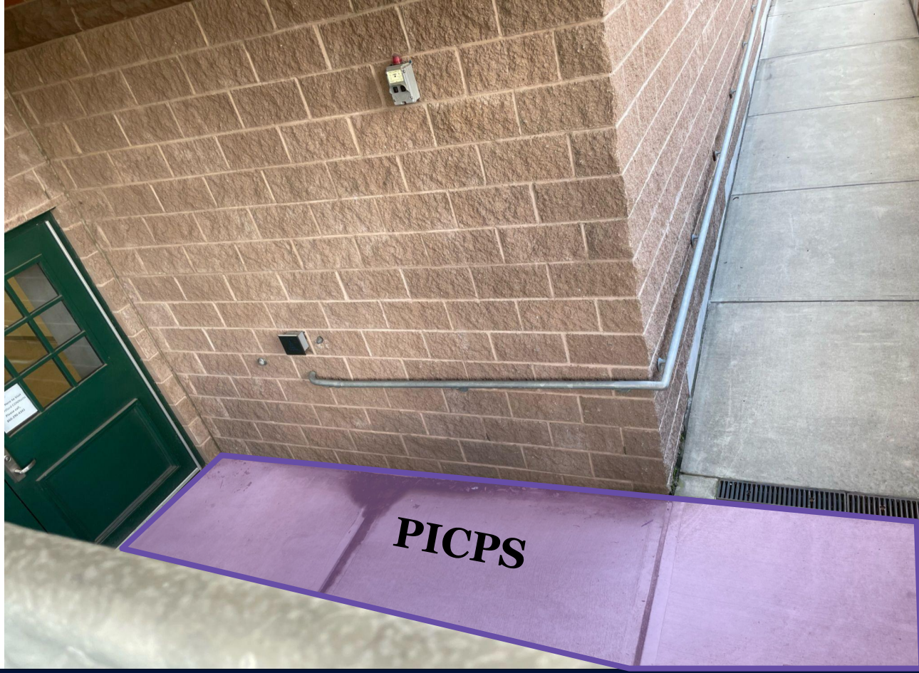
Project #3: PICPs at Raymond Library
