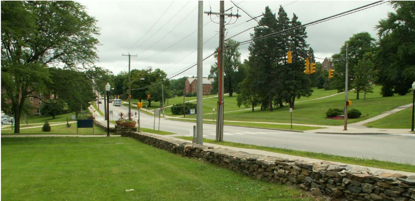
Existing issues along Storrs Road include inconsistent edge treatment and visually intrusive overhead utilities.
