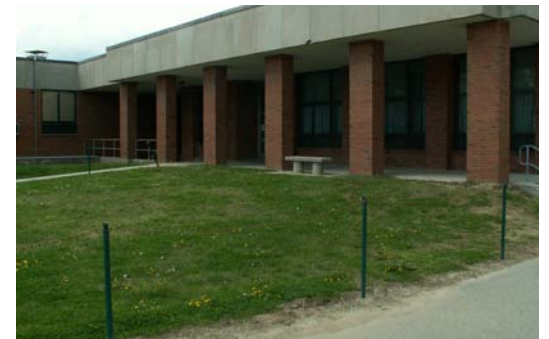
The lawn areas around the Putnam Refectory building should be restored and planted with canopy trees.
