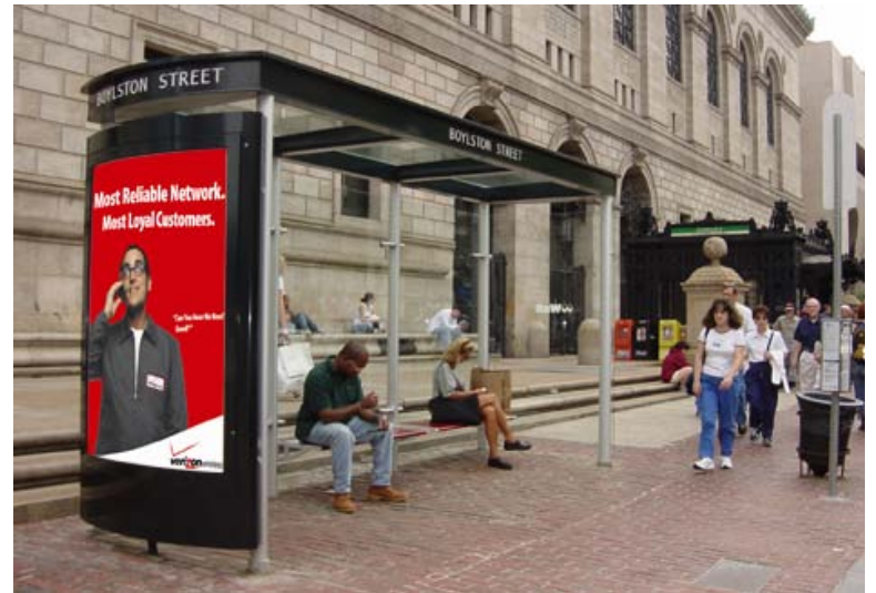
The Boston city standard bus shelter from Cemusa is light and transparent and coordinates with both historic and contemporary architecture.
