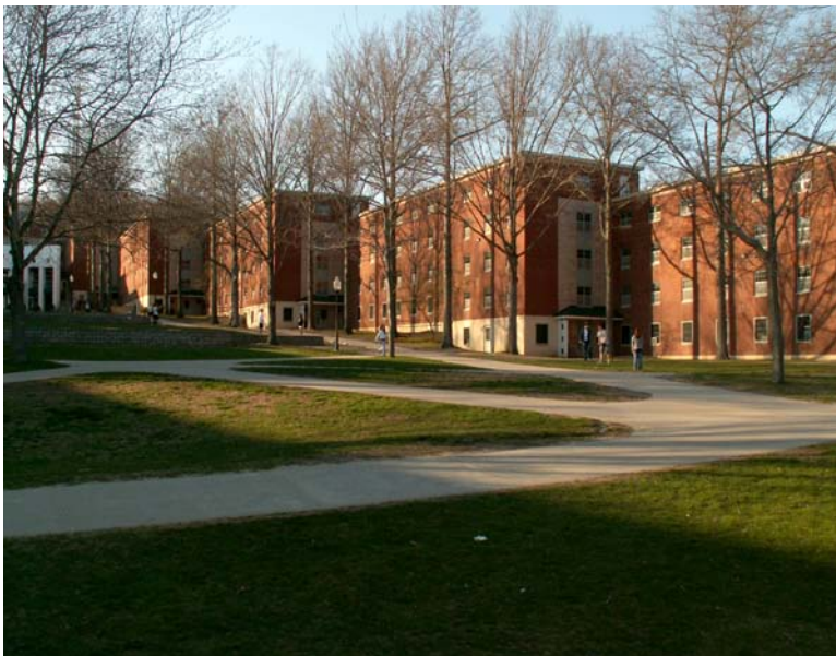
The root zones of the mature canopy trees at North Residence Halls should be protected from foot traffic through the installation of post and chain.
