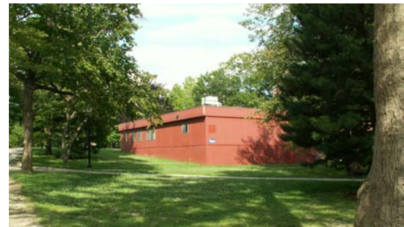
These temporary structures interrupt the carefully arranged composition of buildings and landscape in the historic Lowrie campus. These structures should be relocated and the space they occupied should be returned to naturalistic park
