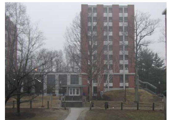
Existing woodland should be protected at Brian McMahon Residence Hall
