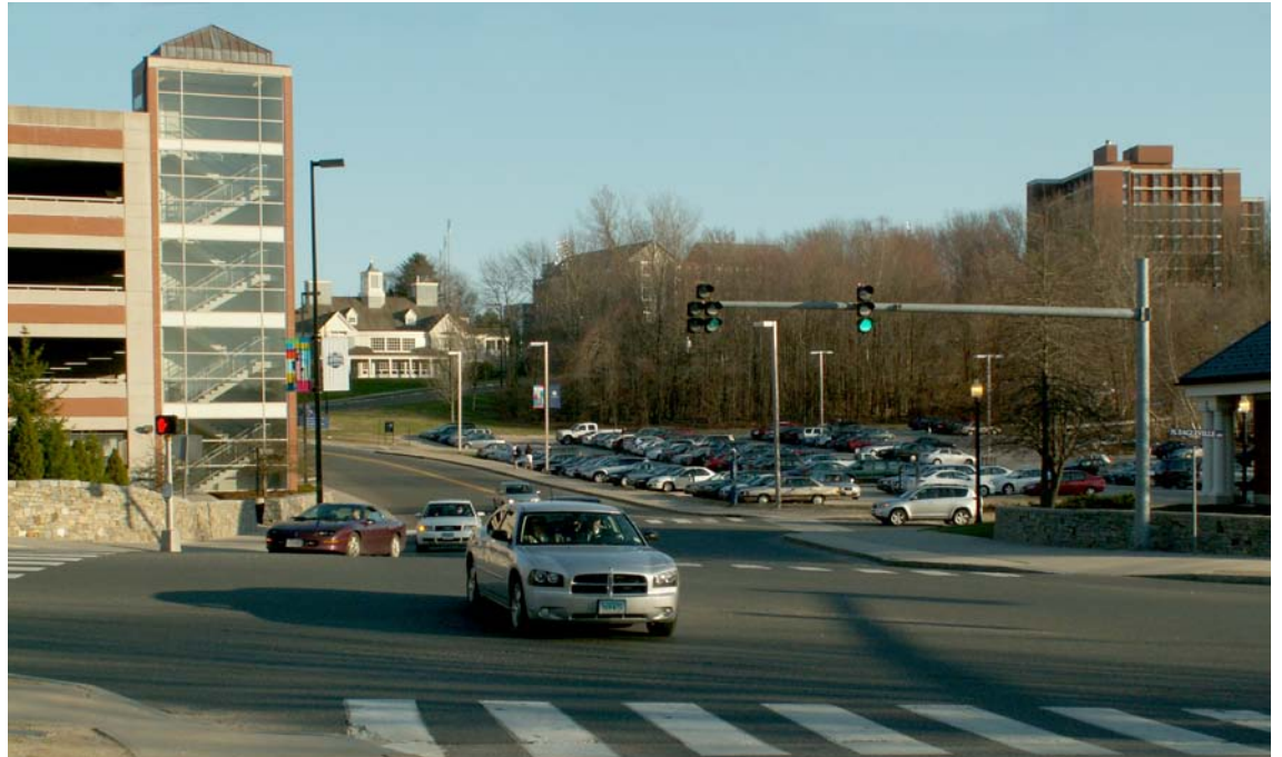
Existing conditions at the intersection of Hillside Road and North Eagleville Road.
