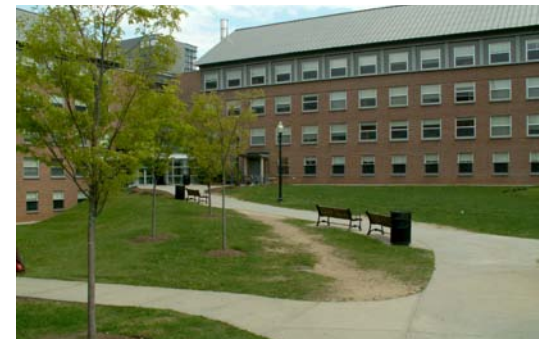
The W.L. Garrigus Suites courtyard requires detailed site design.
