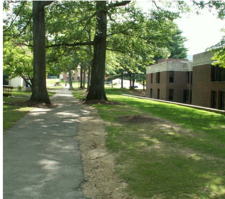
The existing asphalt walks next to the Graduate Residences should be removed and replaced with appropriately sized concrete walks.
