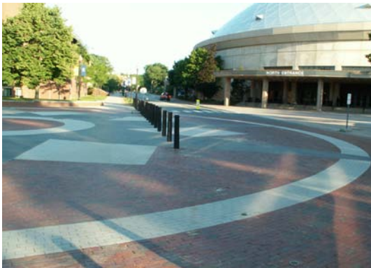
New pavers along Hillside Road should match the existing red brick pavers in the Fairfield Mall seal.
