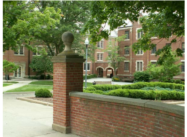
The brick and limestone wall at Whitney Hall is appropriate in scale and character to the adjacent traditional architecture
