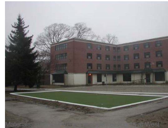
Materials surrounding the courtyard at West
