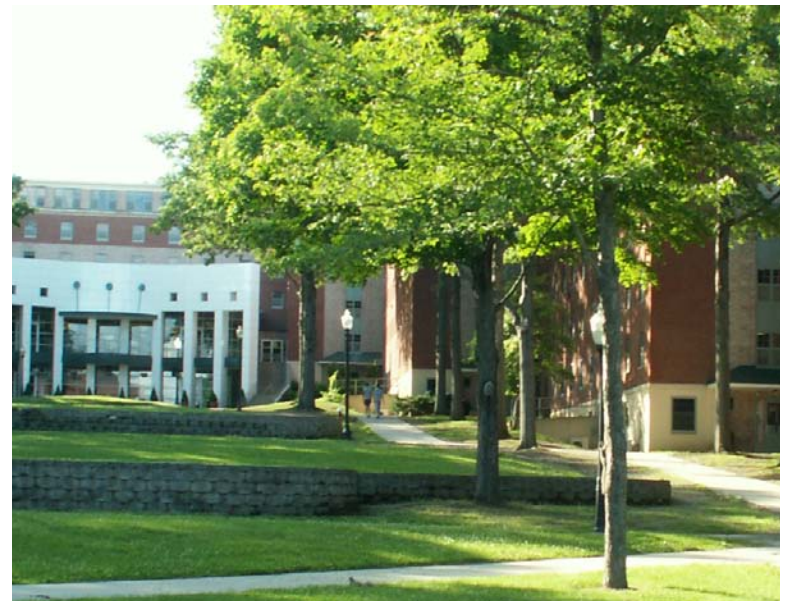
The concrete block retaining walls at the Northwest Residence Halls should be replaced with materials that are more in keeping with the surrounding architecture,
