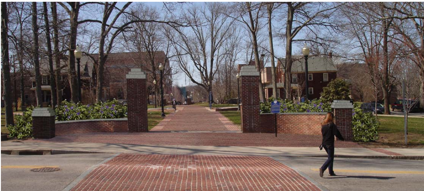
Proposed Academic Way gateway renovation at Gilbert Road
