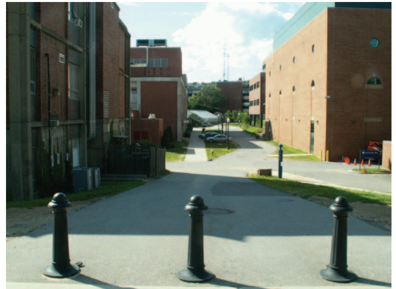
Intersection of Glenbrook Road and Auditorium Road looking towards the Life Sciences Building. The existing service drive and sidewalk should be redesigned as an extension of the Academic Way. The addition of street trees will create a pedestrian scale along the street.
