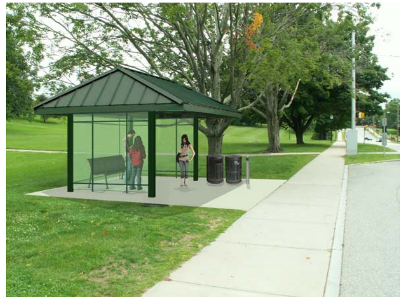
Renovations to the existing campus standard bus shelter include painting the roof a dark green color, and replacement of the brick and plexiglas walls with slim metal columns and tempered safety glass.
