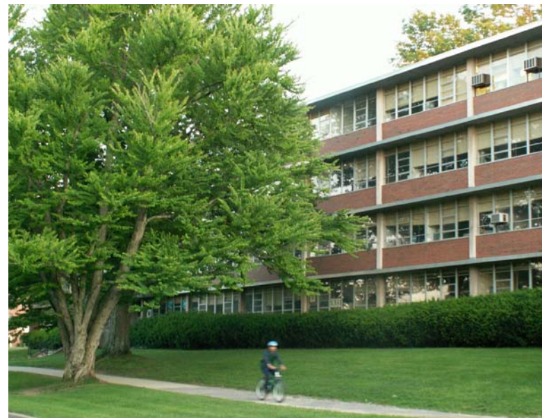
The bold simple foundation planting at the Humanities Building is appropriate to the scale of an institutional building
