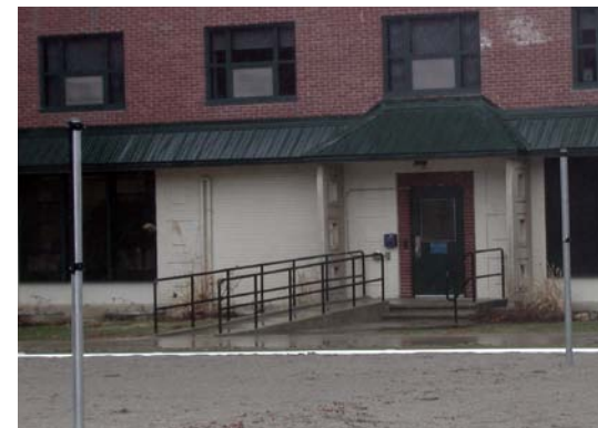
Campus standard stairs and handrails should replace the mismatched entrances at West Campus Residence Hall
