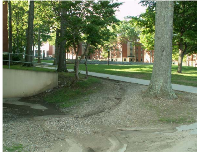
Existing erosion at the North Campus Residence Halls.
