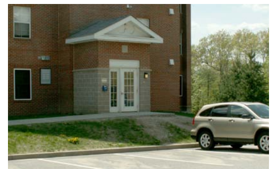
Building entry walks at the Hilltop Apartments should be redesigned with steps and walls to better serve pedestrian circulation and achieve a maintainable condition.
