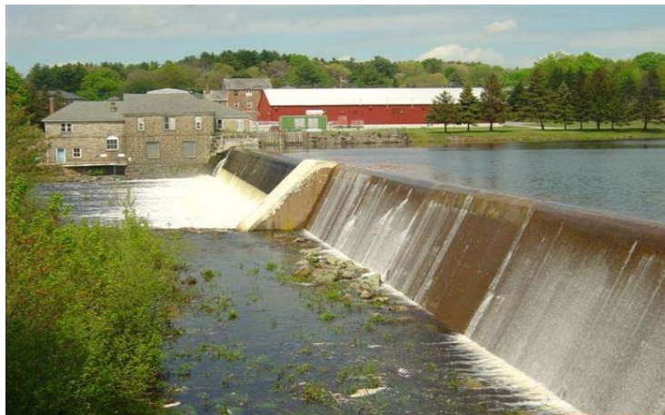
Windham Water Works Facility
