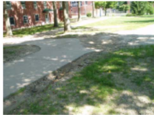
Figure 1. Runoff from quad walkways resulting in erosion (top); Sediment accumulation on walkways and in quad area (bottom).
