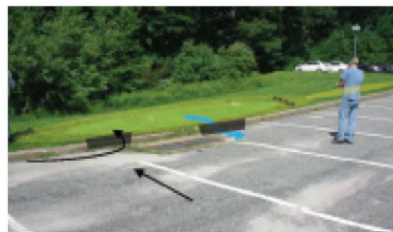
Figure 3. Remove curb along sides of double inlets to allow surface runoff into bioretention area through paved flume with riprap channel. Primary overflow where ponded water "backs up" into existing inlet (blue arrow).
