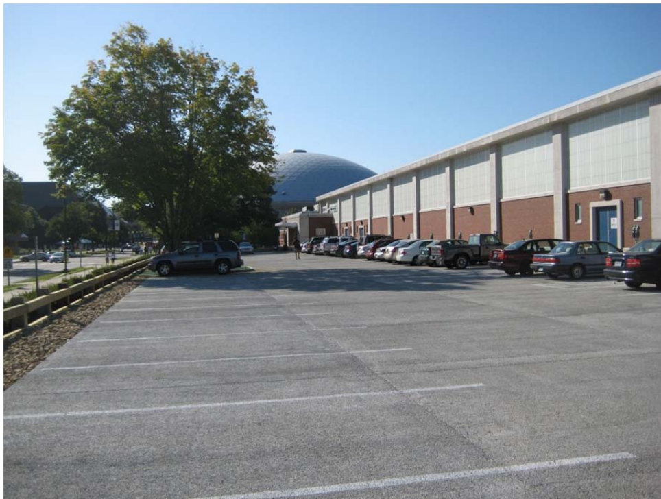
Figure 11. Pervious concrete in front of field house.
