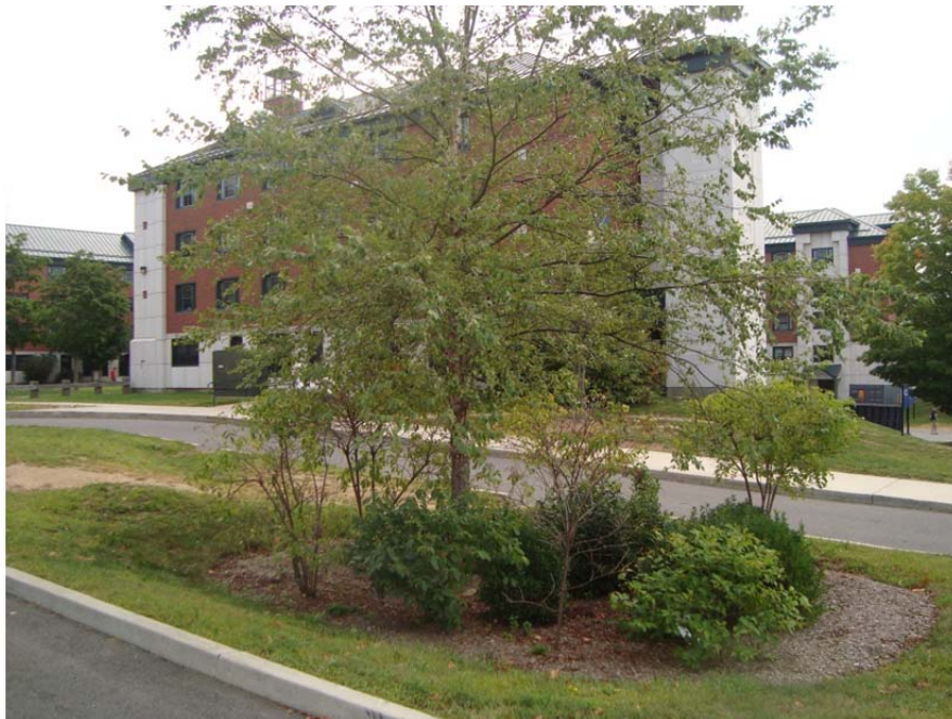
Figure 5. Bioretention by Towers dorms.
