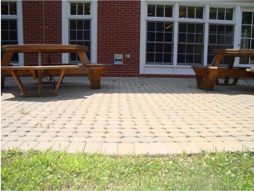
Figure 9. Pervious pavers at Lakeside Apartments.
