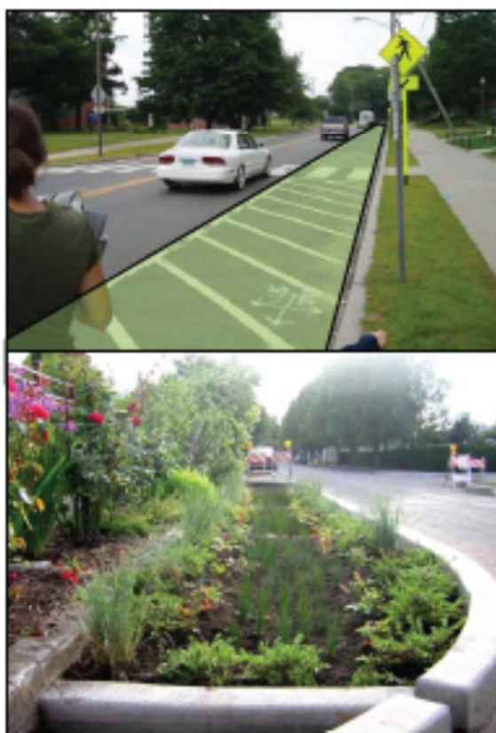
Figure 2. Remove pavement along existing road shoulder to edge of existing curb (top). Example street planters with curb cuts from Portland, OR (bottom).
