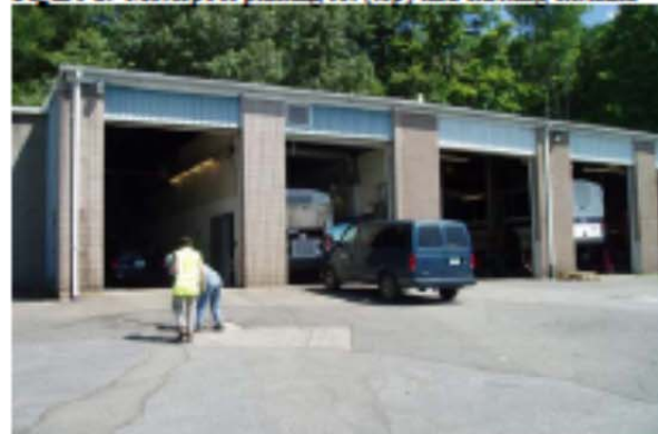
Figure 2. Motorpool parking lot (top) and existing external
