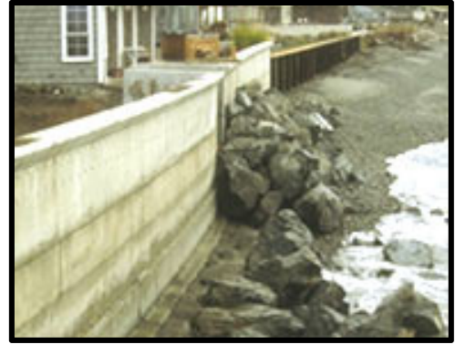
Narrowed beach in front of a bulkhead. Photo: WA Department of Ecology.
