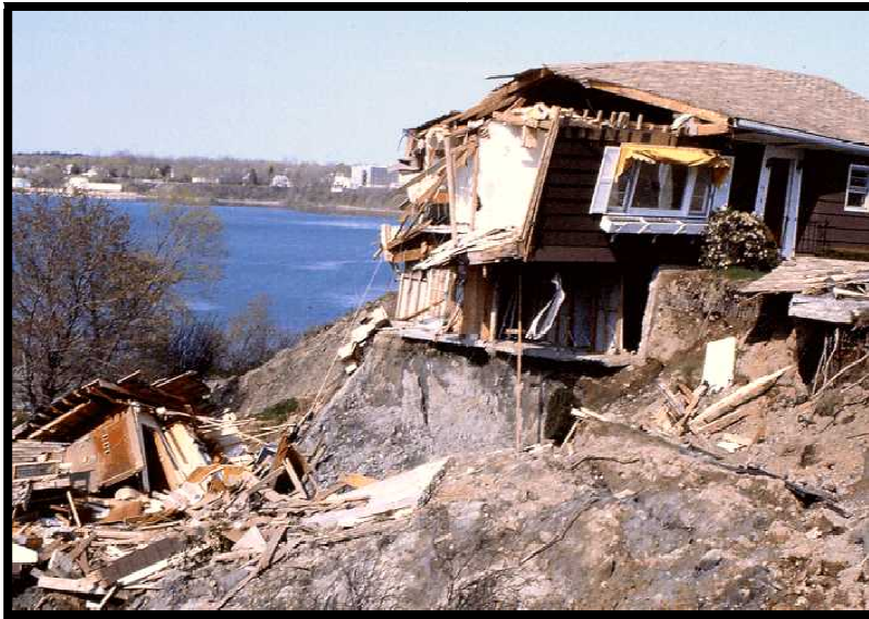
A clay bluff on the north shore of Rockland Harbor failed in 1996. This landslide formed a new scarp about 200 feet landward of the original top of the bluff in just a few hours. Two homes were destroyed. Photo: Maine Department of Agriculture, Conservation, and Forestry.
