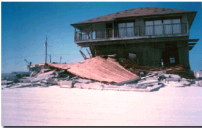
Damage from Opal. Photo: FL Department of Environmental Protection
