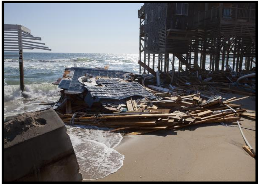
Rodanthe, North Carolina, Sep. 3, 2011. Hurricane Irene destroyed homes and eroded beaches to the point that the waves now reach under this elevated house.
