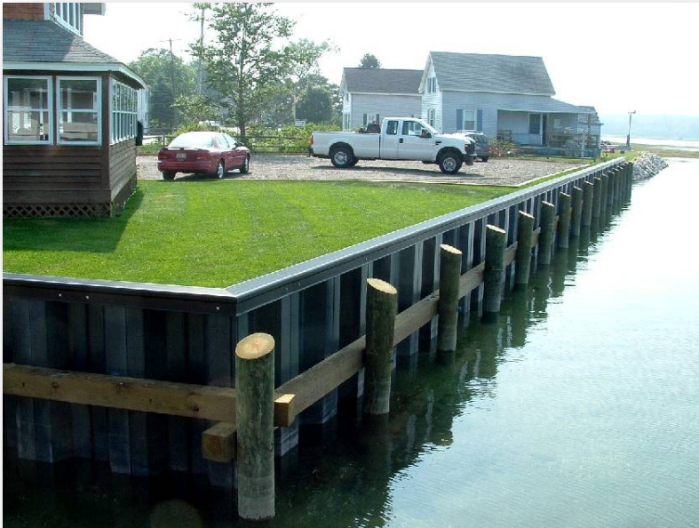
Timber or Sheet Pile Bulkheads
