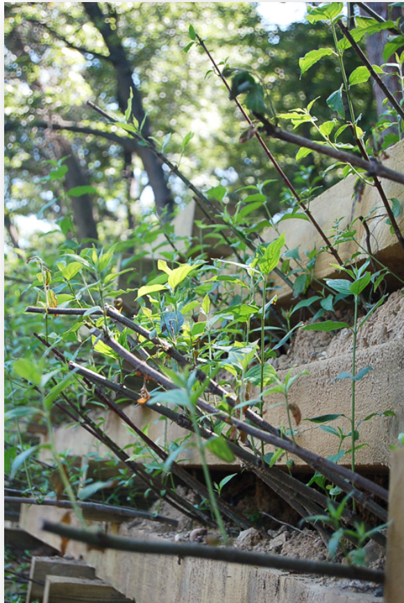
Live Crib Walls
